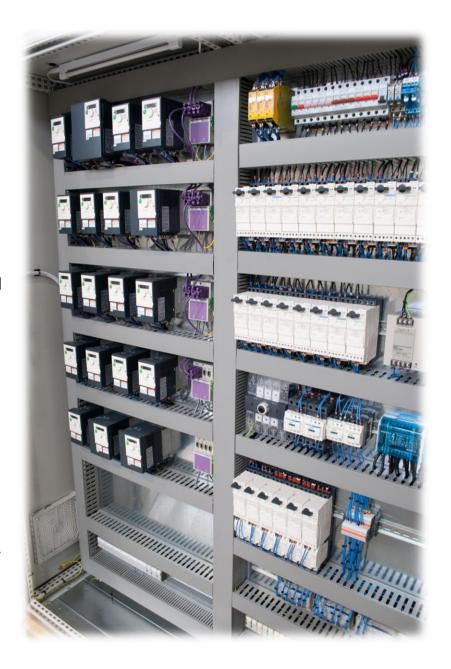
The Control Panel itself is used to control a large product handling system made up of 26 motors, various conveyors, and a large carrousel unit. The system status and control is
