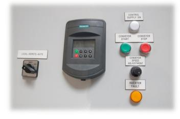
control panel. The large 55Kw inverter is controlled from the front of the enclosure via a keypad with integrated display. All speed adjustments are made from a potentiometer also mounted on the front of the enclosure. As with all our large floor standing control panels, both sections are illuminated to aid installation and testing on site. The panel is fully tested in our workshop where the inverter parameters are also set-up. The control panel also
