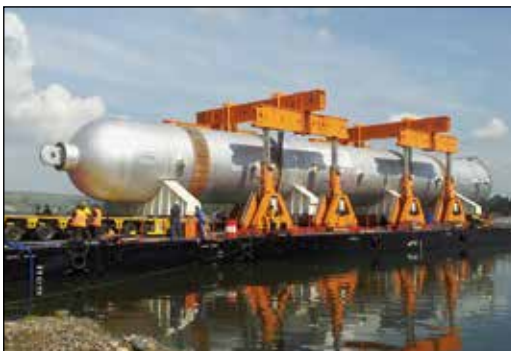
◀ Two SBL1100 gantry systems lifted the 1300 ton hydrocracker off the barge onto a SPMT Self-Propelled Modular Transporter.
