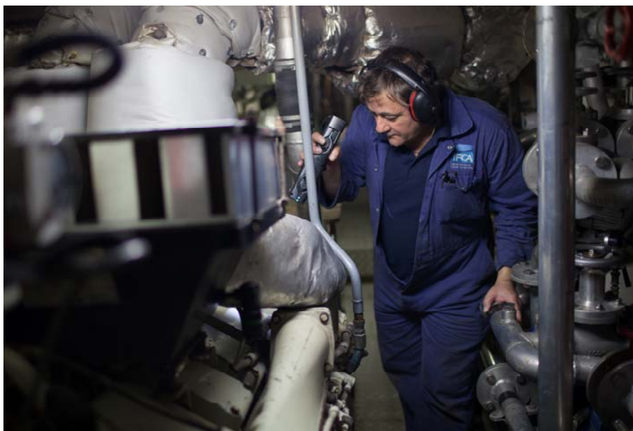
John Keast inspecting Saint Piran's engine room (Copyright Simon White)
