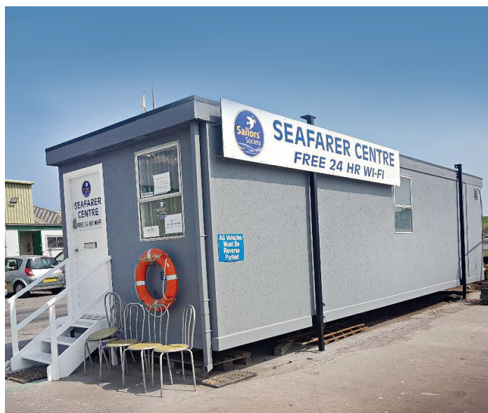
The refurbished Montrose Seafarers' Centre
