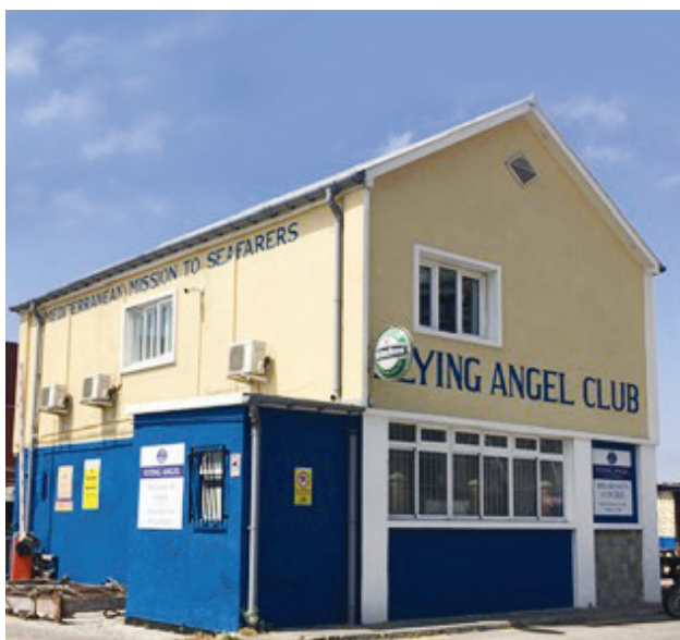
The interior and exterior of the Flying Angel Club were repaired after damage from water ingress and years of exposure to the elements
