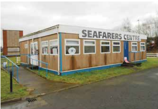
Before and after photos of the refurbished Grangemouth Seafarers' Centre
