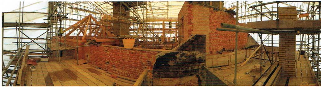
←← Oulton Hall Undergoing Reconstruction
