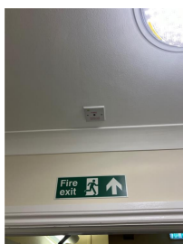
Fire escape route indicated
