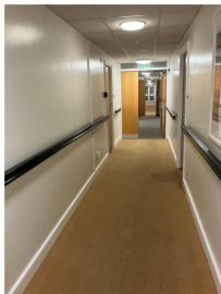
Handrails on corridors
