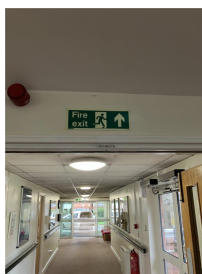
Fire escape route clear signage
