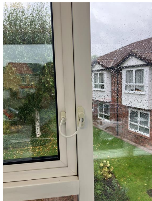
Window restrictor first floor
