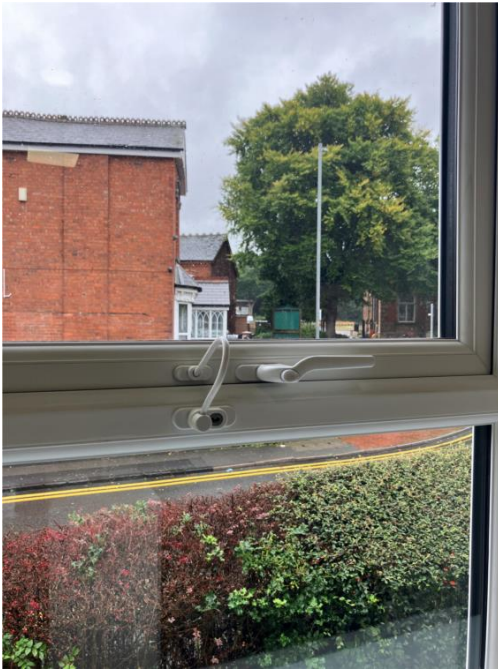
Window restrictor first floor
