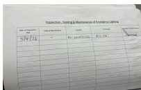
Emergency lighting monthly tests
