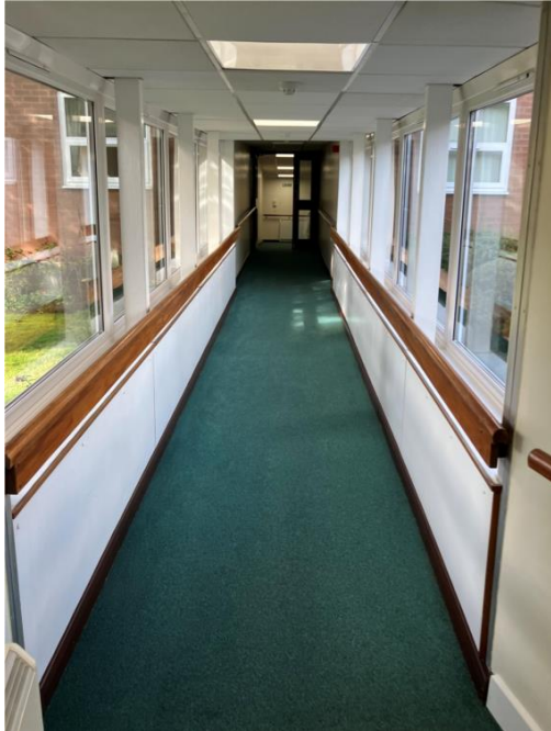
Hand rails on corridors
