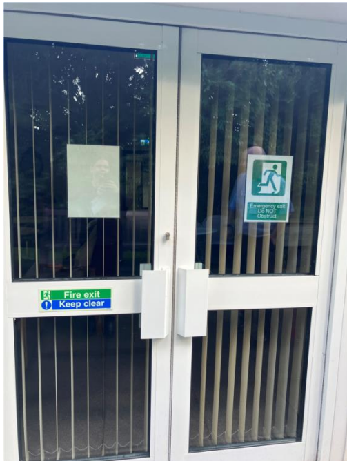
Fire Exit - clear signage on both sides of door
