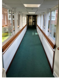
Hand rails on corridors
