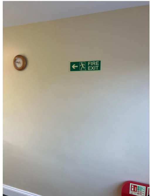
Fire escape route indicated
