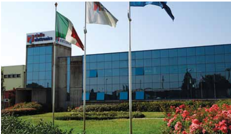
Riello Elettronica: the headquarter.
