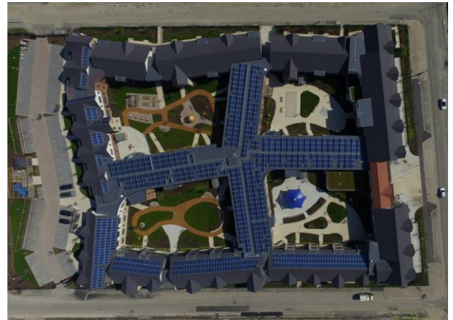
Drone Image of Completed Works:
