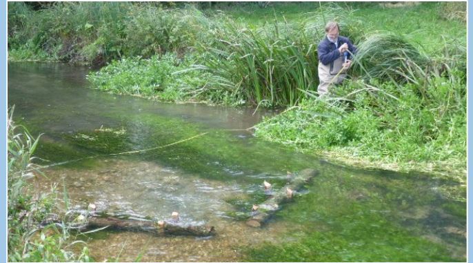
V-structure to promote bed scouring
