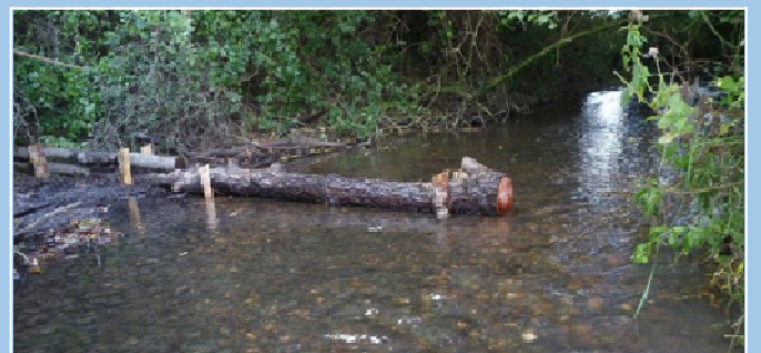
Log deflector to accelerate the flow
