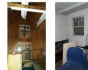
INTERIOR OF PAVILION & CHANGING ROOM
