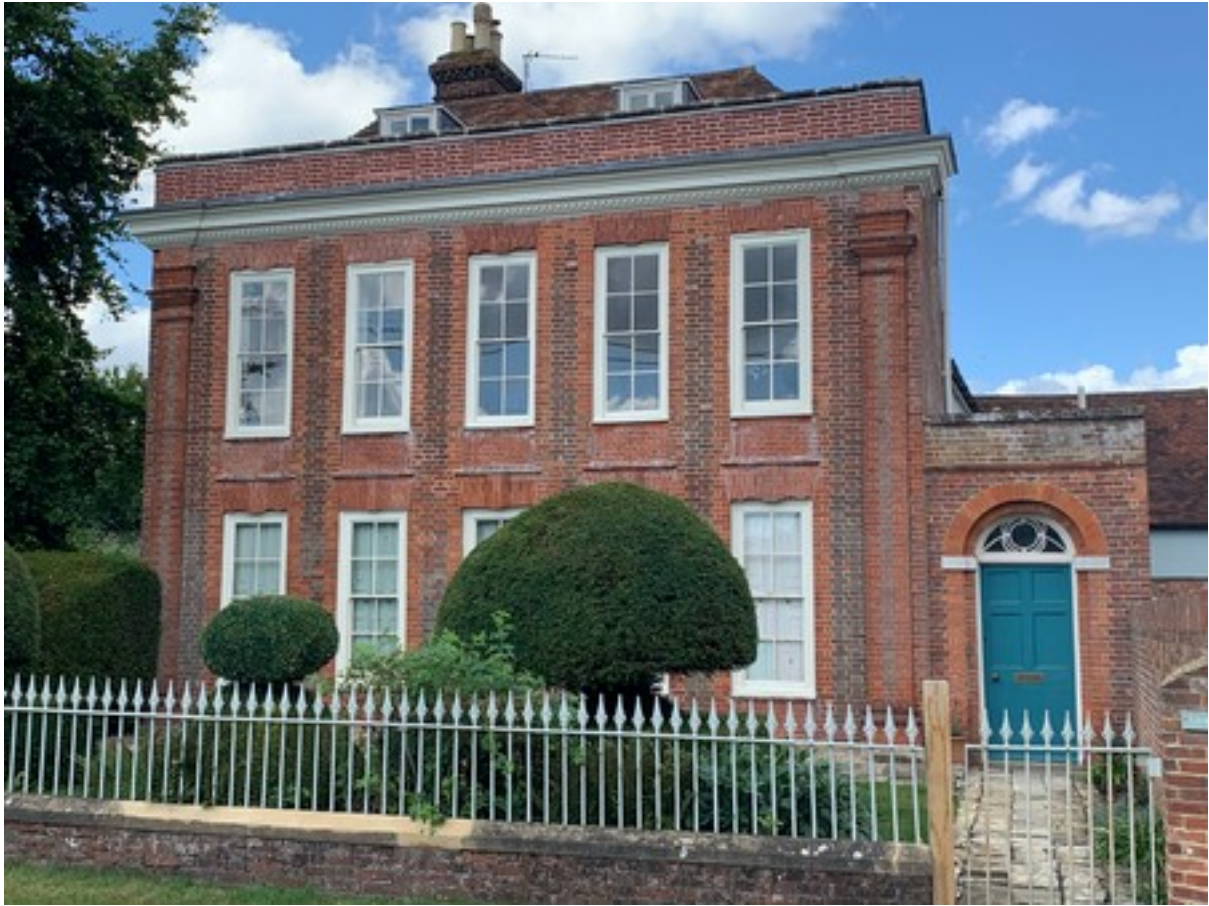
Following front façade restoration 2019
