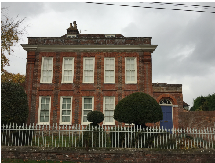
Prior to front façade restoration
