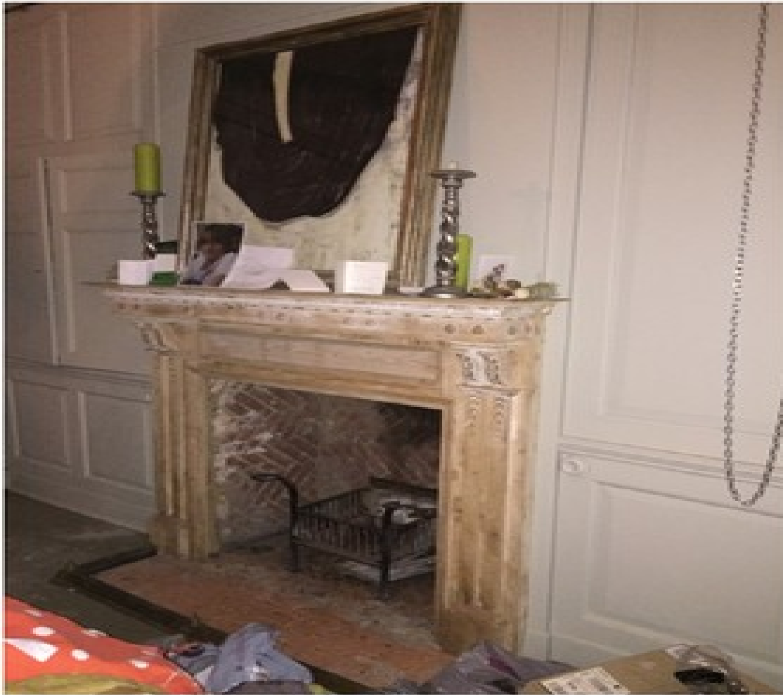
10. Phase 2 panelling and fireplace ground floor
