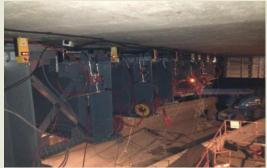
Once the defined loads and displacement was achieved, all the hydraulic jacks were mechanically "locked-off" by the screw-ram locking collar. Once completed, Hydra Capsule installed custom-made grout bags which were inserted at each bearing location and inflated by our grout pump, to wedge the gap.
