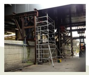
In addition, once all the piers had all the remedial works and bearing replacement completed. Hydra Capsule re-attended site to de-energise and transfer the existing loads back-trough the newly installed elastomeric and fixed bearings.
