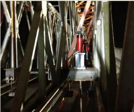
The hollow ram cylinders were installed using high-strength threaded-rod bar, which supported the bridge-deck underneath and supported the bridge top deck. All supported off an independent temporary frame.
