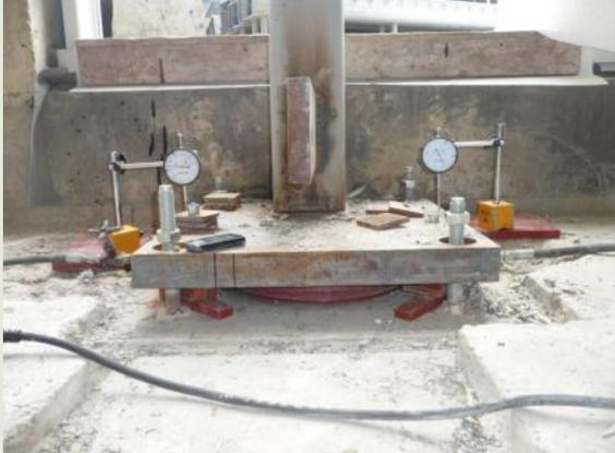
The grout transfusion operation consisted of a skilled trained jacking team to accurately transfuse Temporary fluid (water / oil) from the flat jack, and inject cementitious grout into the flat jack capsule.
