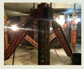
Prior to the lifting operations, all the supporting walls and columns were required to be diamond-cut / drilled free of the main structure. This consisted of installation of a complete steel prop arrangement, on each floor to suit the geographical of the building restraints. The 30 number jacks were then installed and fixed on the top of the prop. Which in turn, were pre-loaded for allowing hydro-cutting remedial works to commence and be completed.
