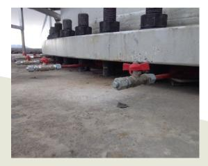
In addition, Hydra Capsule were contracted to carry out flat jack(s) grout transfusion operations for permanent installation. The works were completed under "live conditions". Monitoring movement, pressure / load continuously, With accuracy of 0.25mm.
