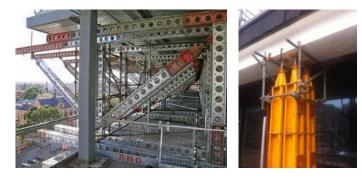
With a comprehensive range of soldiers and accessories, the temporary propping system can be assembled into:
