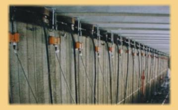
The system accommodates all our electronic instrumentation to be interlinked as one circuit to a central-control system, which formulates the computer control system to monitor each jacking position with movement stroke sensors, pressure transducers and electronic solenoid flow-control, regardless of the load and quantity of jacks within a circuit.
