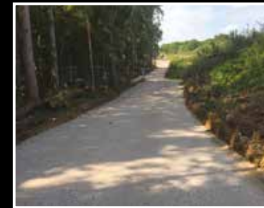
Stage 4. Surfacing can be laid and trafficking can commence in 24hrs in the summer months and 48hrs in the winter months.
