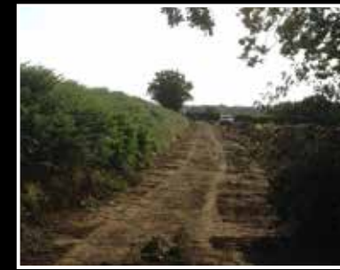
Stage 1. Work site prior to stabilising commencing. Effective stabilisation was achieved despite adverse conditions.
