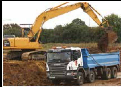
1. Material excavated from site
