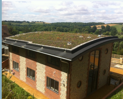
Thompson house from the back with stunning views of the landscape and the sedum roof
