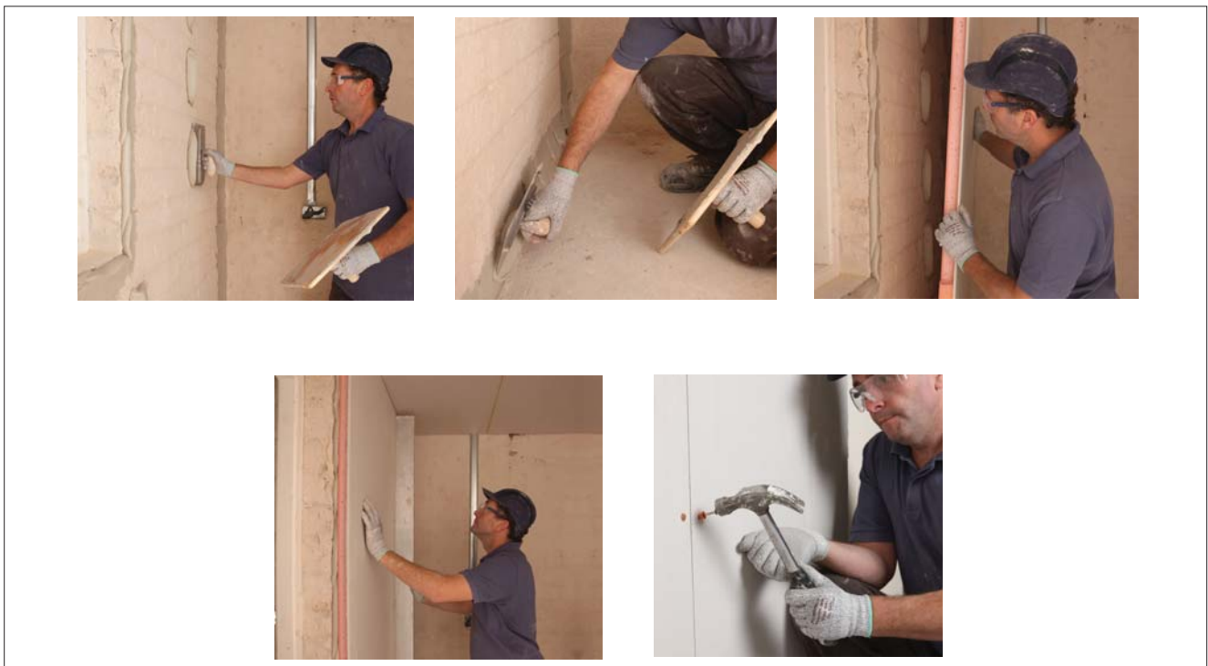
Figure 3 Drilyner TL installation details
