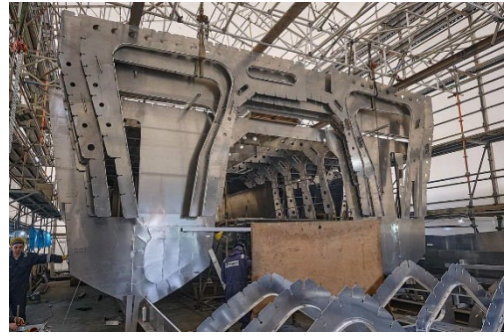
Framing & Plating May 2024
