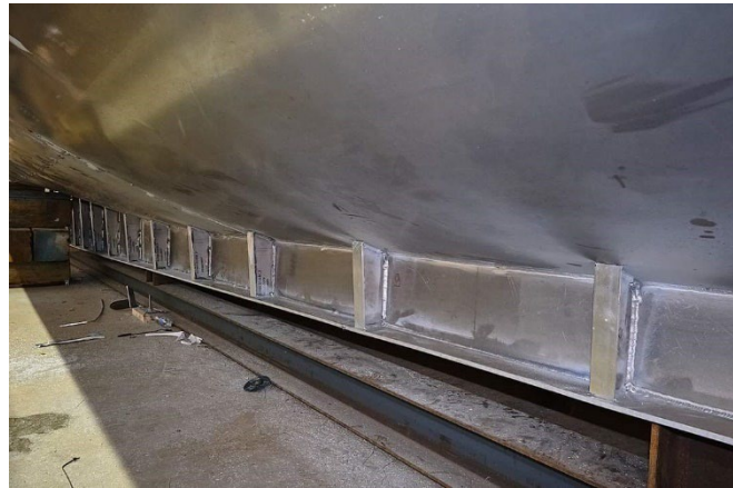
Hull plating May 2024
