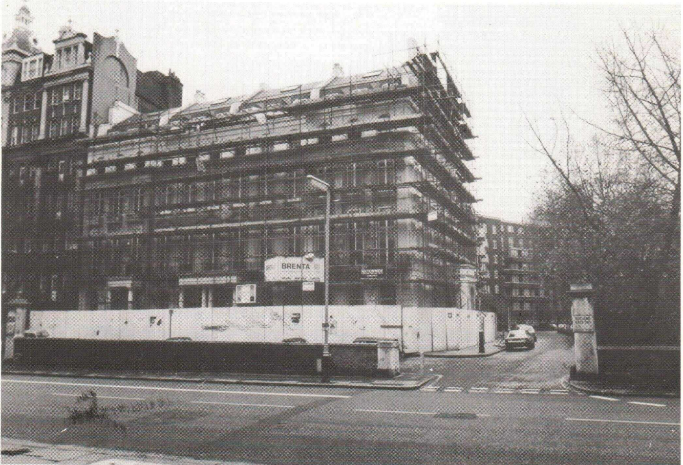
The eastern entrance to Rutland Gate where a renovation is taking place
