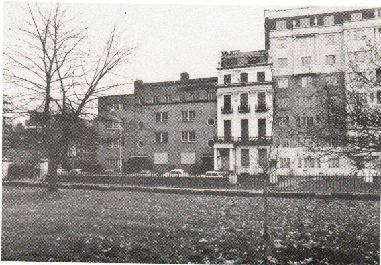
The western entrance to Rutland Gate where a development is envisaged
