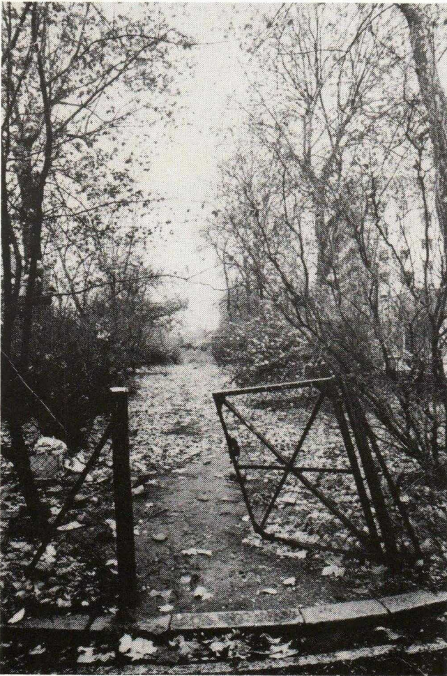
The dilapidated Upper Gardens, Rutland Gate.
