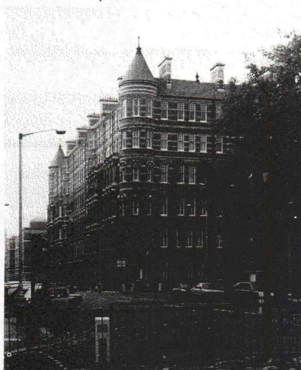
Albert Court: roof line saved.
