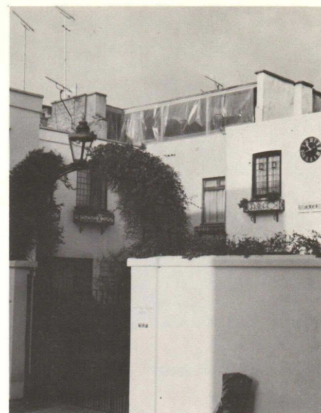
Addition to Box Cottage.
