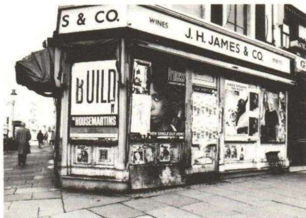
Dilapidated state of 130 Brompton Road, despite planning permission having been granted some months ago.
