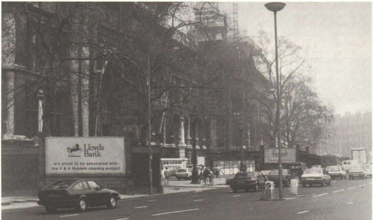
Proposed temporary walkway during work at the V & A showing sponsorship advertising.
