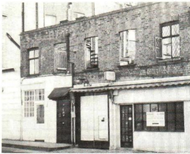
1-3 Cheval Place in course of demolition.
