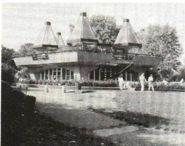
The Serpentine Restaurant which is being demolished.
