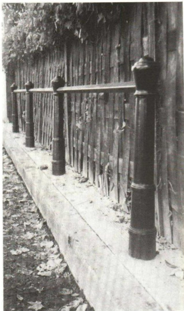
Before: The sad relics of the original hitching posts in Rutland Street. After: The restored hitching posts and railings cast from the one remaining original.
