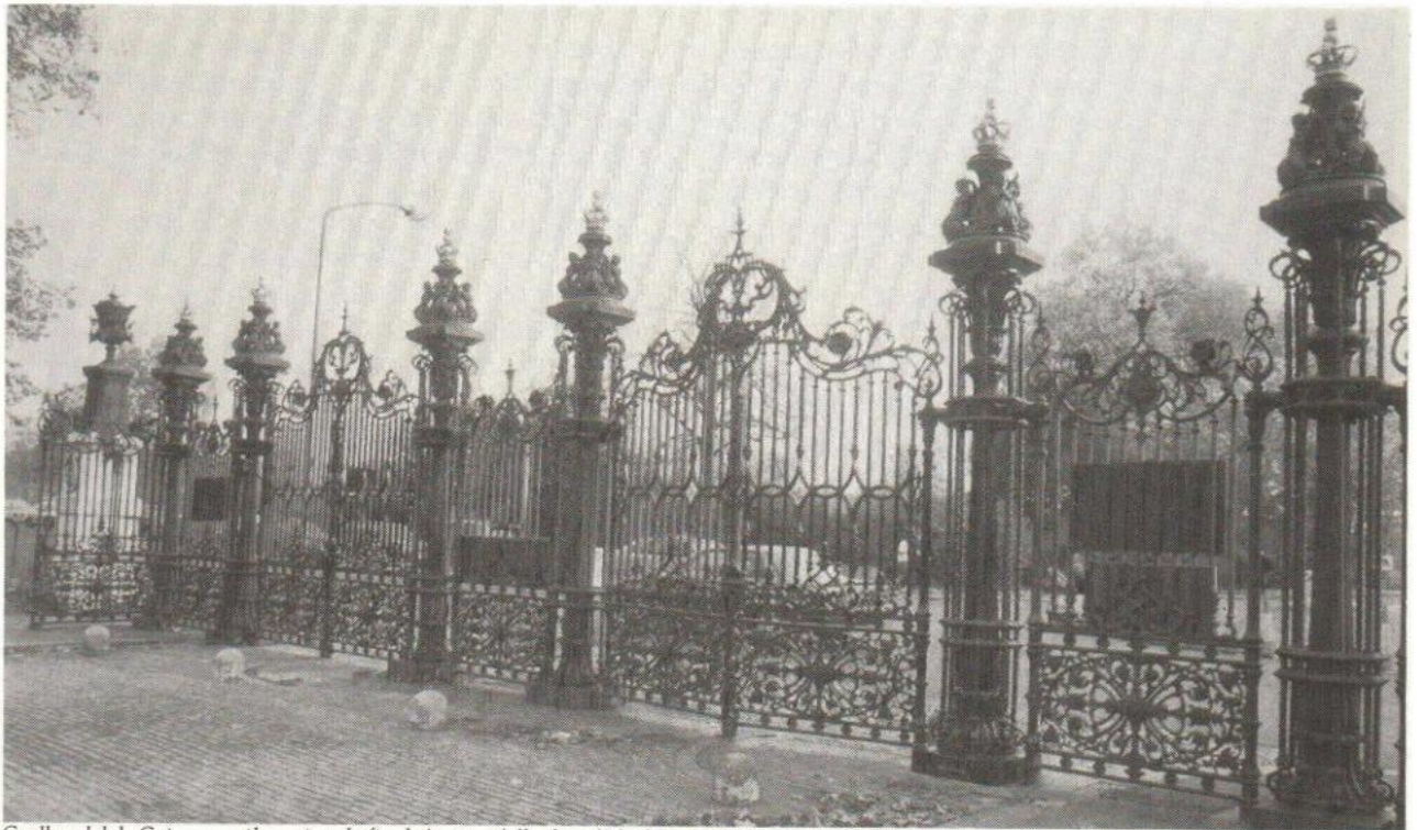
Coalbrookdale Gate, recently restored after being partially demolished in a traffic accident in 1988. It takes its name from Abraham Darby's Coalbrookdale Foundry, established in 1709.
