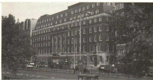
Agriculture House, a post war building which would be demolished in a new scheme.
