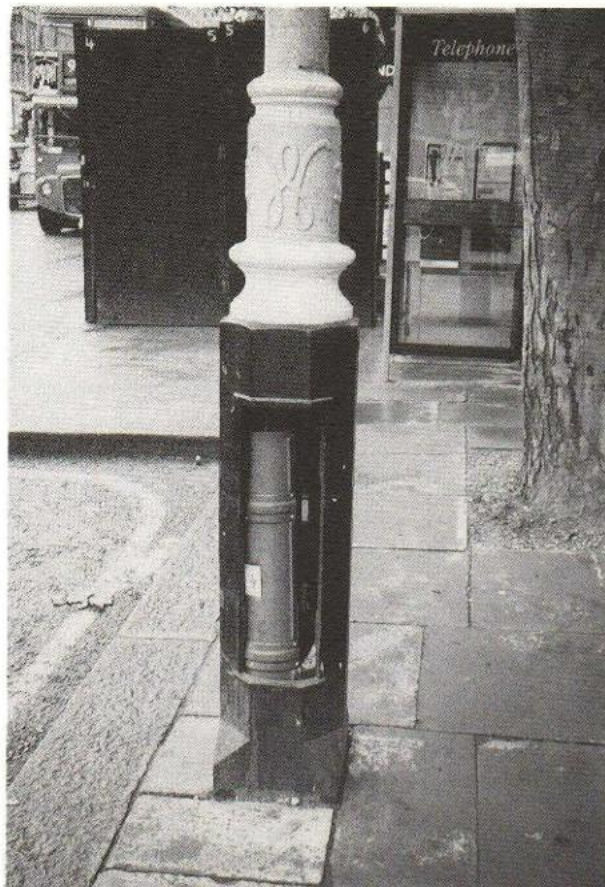
Recurrent problems: broken paving (above) and exposed wiring (below).
