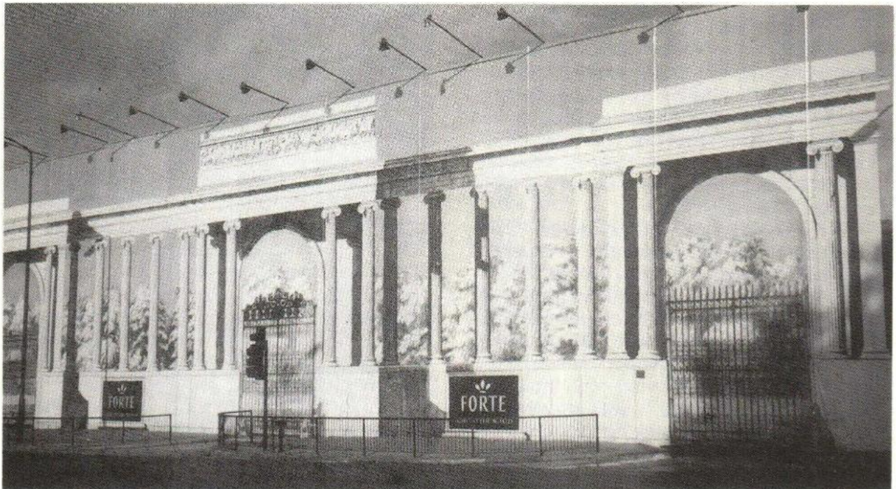
Not the Decimus Burton Screen, but an imaginatively conceived sponsored painted canvas hoarding, hiding unsightly scaffolding during repairs.
