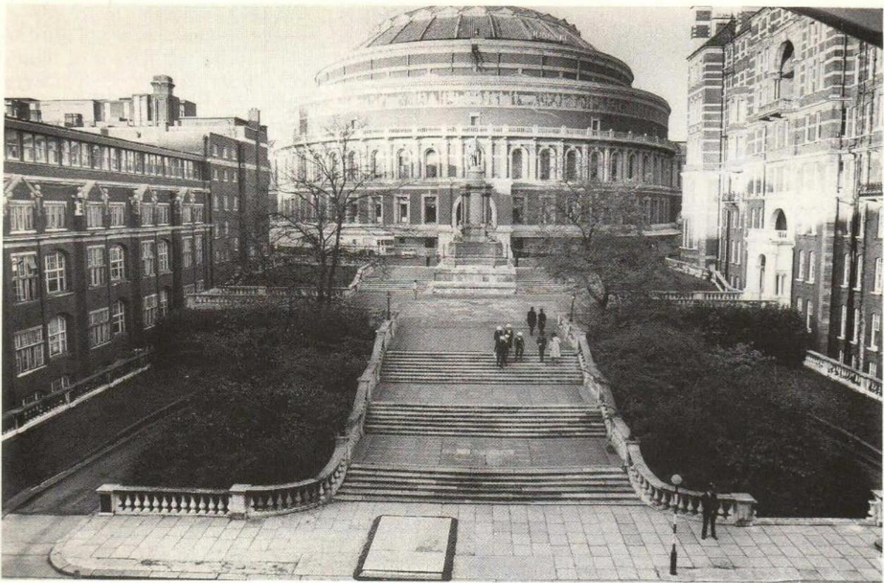
The steps to the Albert Hall from Prince Consort Road, which have been acquired by the Albert Hall management, making possible a development plan which should benefit ticketholders and local residents. (See page 16.)
