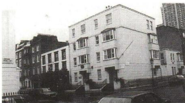
Buildings due to be demolished and replaced with single family homes.
