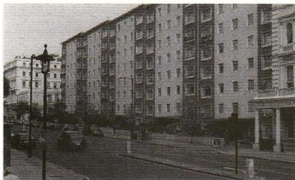
Montrose Court, built in the mid 50's. The extra storey will be set back from the front (see Appeals)..
