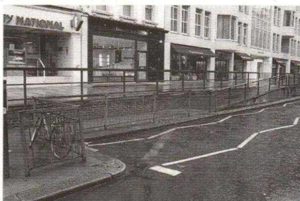
Split level pavements in Brompton Road would benefit from re-landscaping. New more elegant railings would enhance the whole Knightsbridge and Brompton Road thoroughfare.
