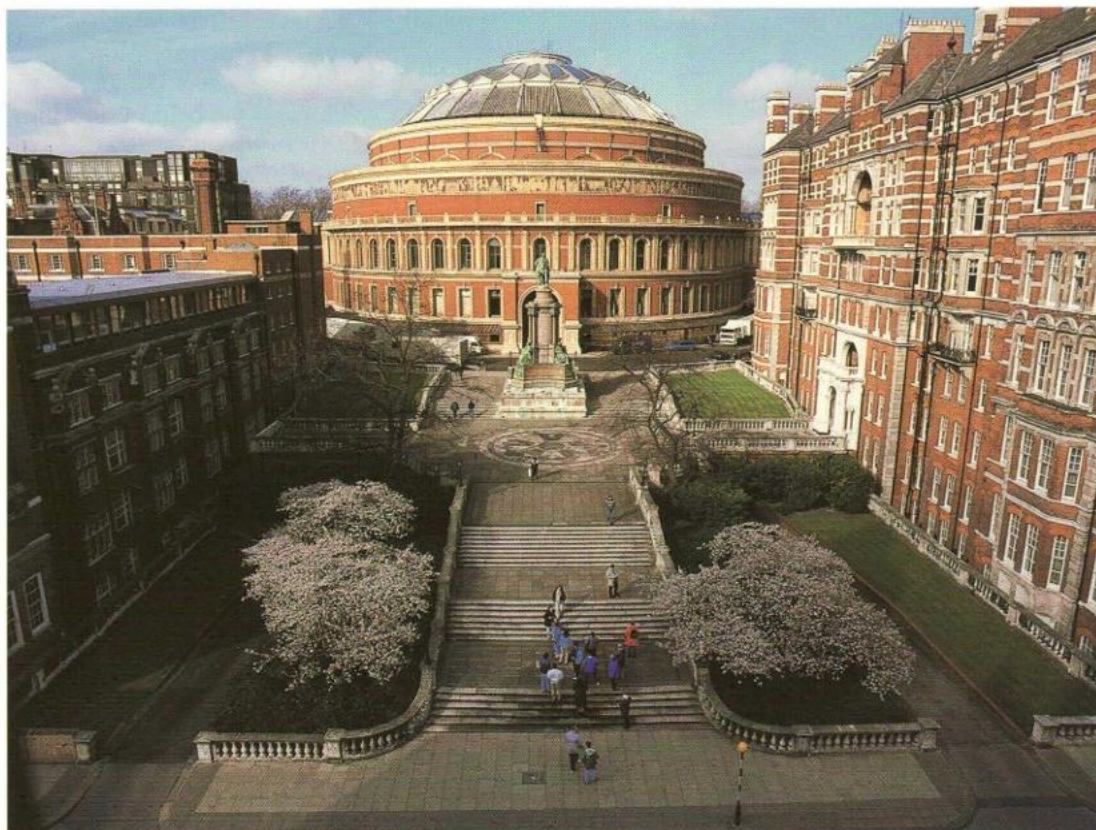
The Royal Albert Hall: South Porch and steps.
