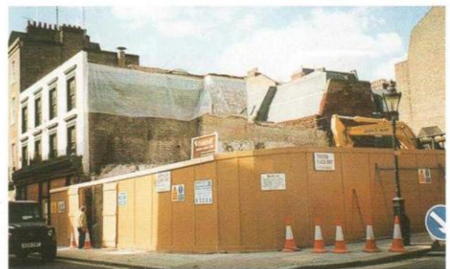
44a & 44b Montpelier Square, formerly the Omani Embassy, is being rebuilt as a single private house.
