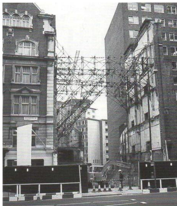
Part of the Normandie site being cleared. Will buildings operations begin soon?
