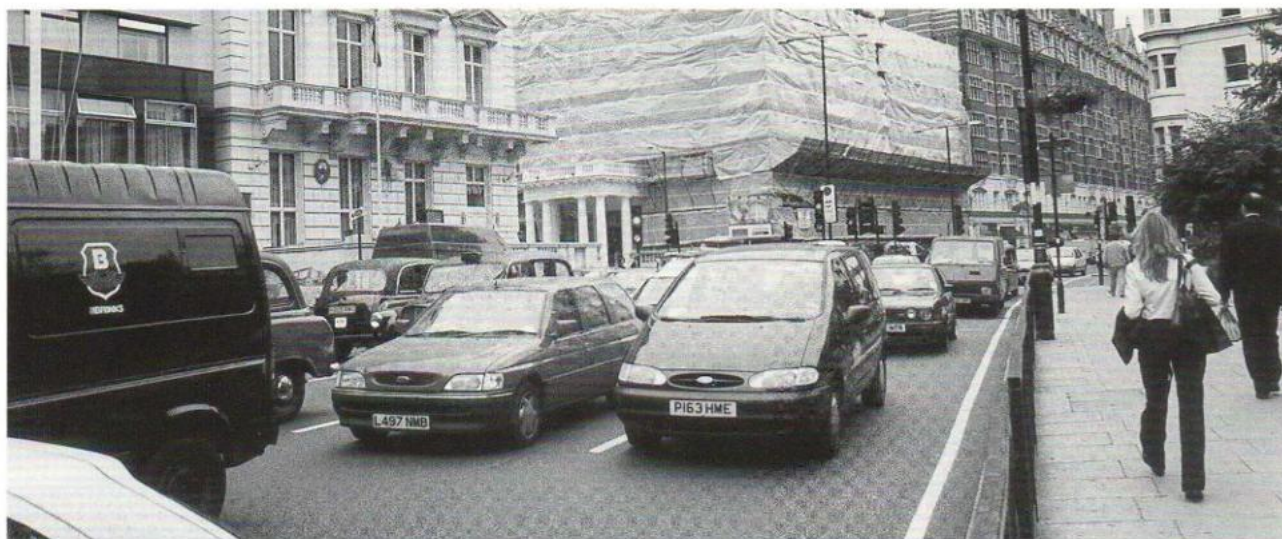
The French Embassy after many years of neglect - a thorough clean and refurbishment due to be completed before Christmas.
