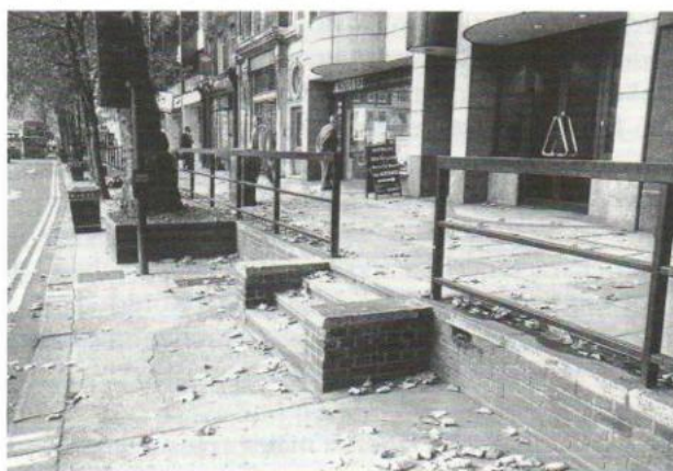
Below: The pilot project. The split level pavement between Montpelier Street and Cheval Place.
