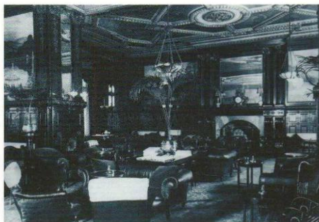
Far left: The newly refurbished lobby.
