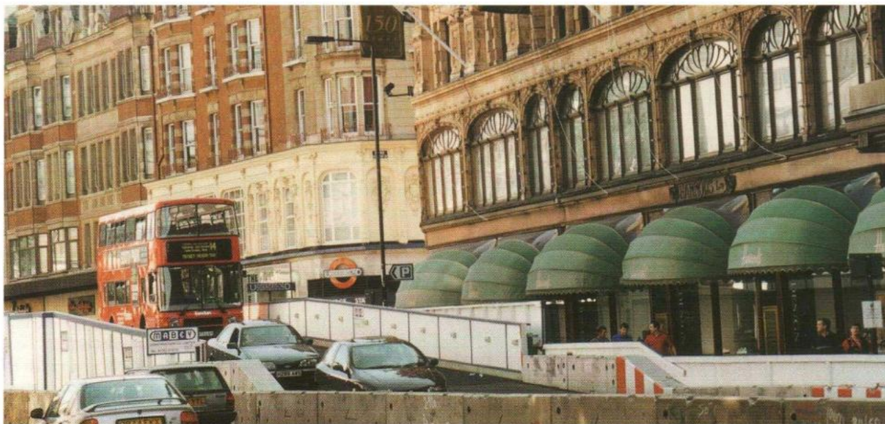
Hans Crescent, closed during improvements to Knightsbridge Tube Station.
