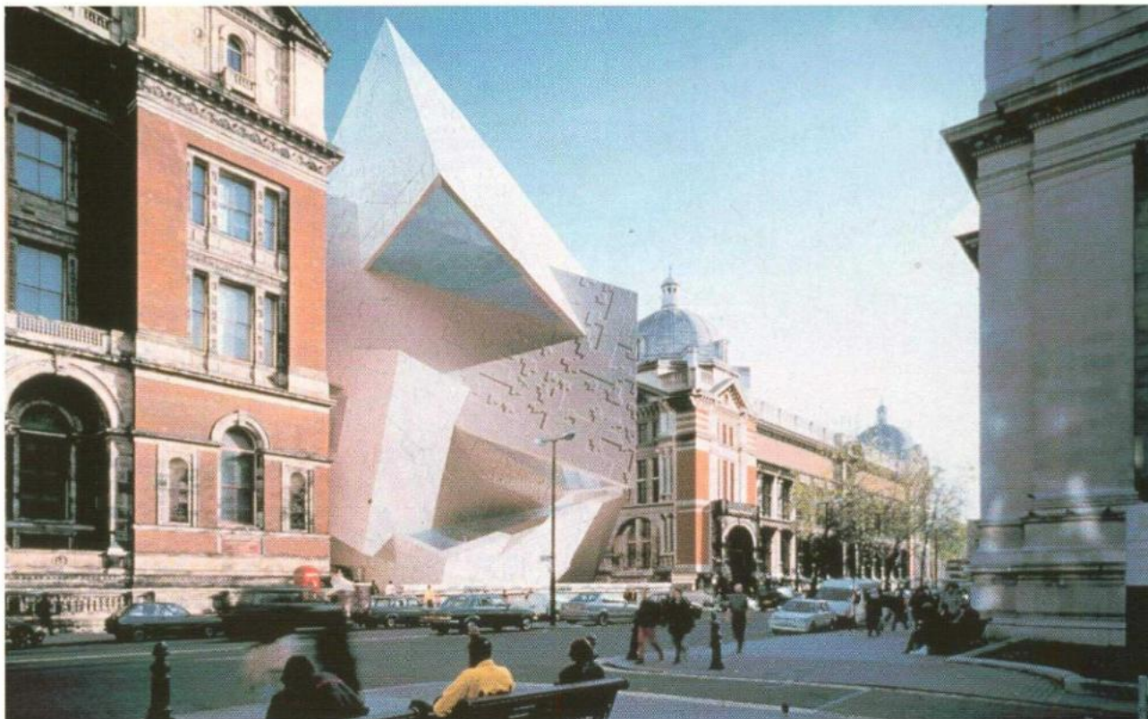
View of the Spiral from Museum Lane looking down Exhibition Road.
