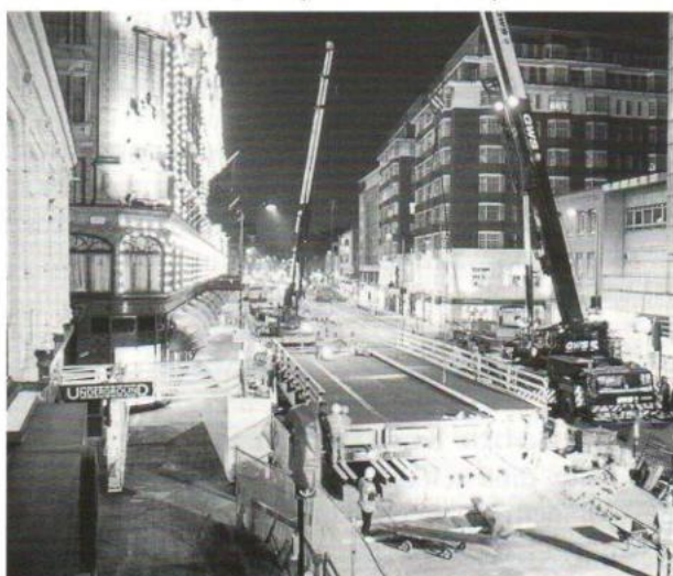
The bridge along Brompton Road to allow excavation below.
