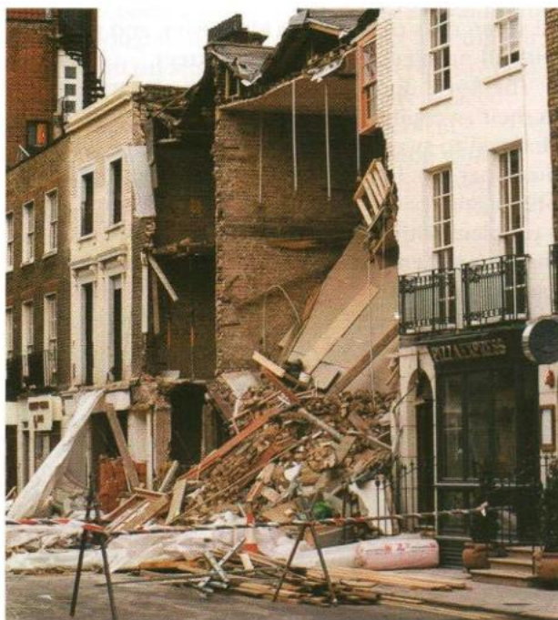
The collapse of two houses in Beauchamp Place during building works at the end of 1998 necessitated the introduction of a one-way system. Coinciding with the complete closure of Hans Crescent during works to Knightsbridge Tube Station, this had an unfortunate knock on effect in the neighbouring residential streets.
