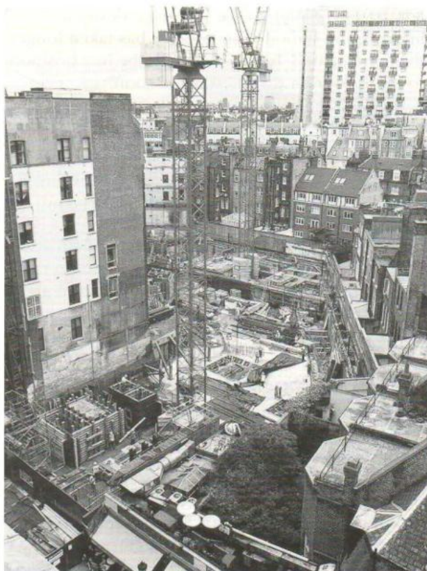
Crown Court site - building work in progress illustrating the complexity of the scheme.
