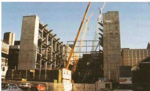
The Wellcome Wing under construction.
