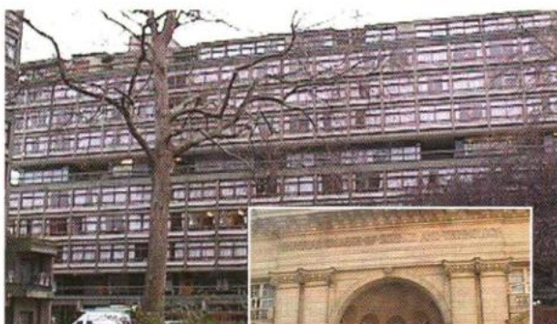
Above: Southside Halls of Residence, built in the Sixties.
