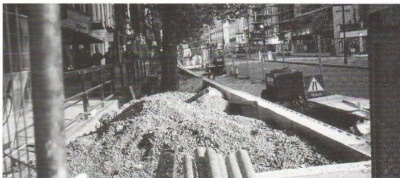
Phase 1 - Work in Progress
