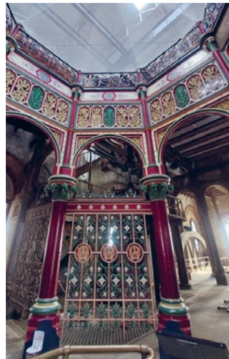
Ornate cast-iron work at Crossness Pumping Station
