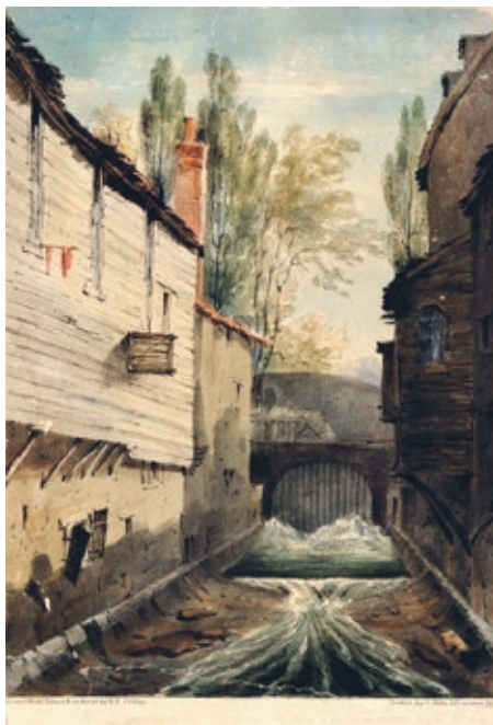
Hand-coloured lithograph by Giles Firman Phillips of the 'Bayswater' (another name for the Westbourne) flowing out of the Serpentine in Hyde Park, into Knightsbridge before it was disconnected from the Serpentine and culverted in 1834. This was roughly the location of the original medieval bridge.
