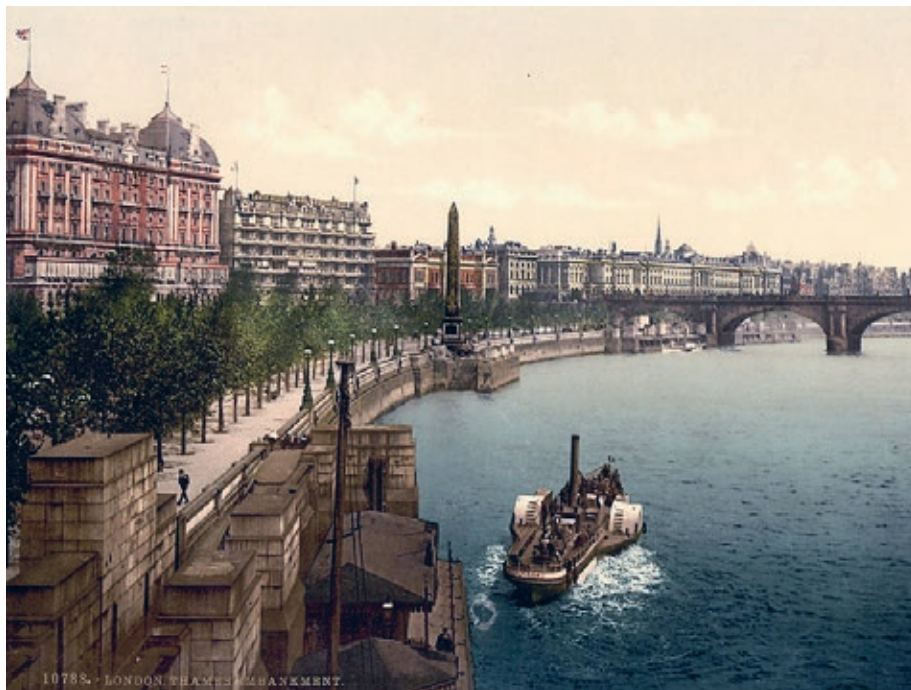
A postcard from the 1890s showing Bazalgette's Thames embankment. The embankment narrowed the river so that it flowed more strongly and also avoided destroying Londoners' properties to house the main interceptor sewers. In addition the embankment replaced much of the river's foreshore which collected waste, providing a modern, sophisticated face for the Thames
