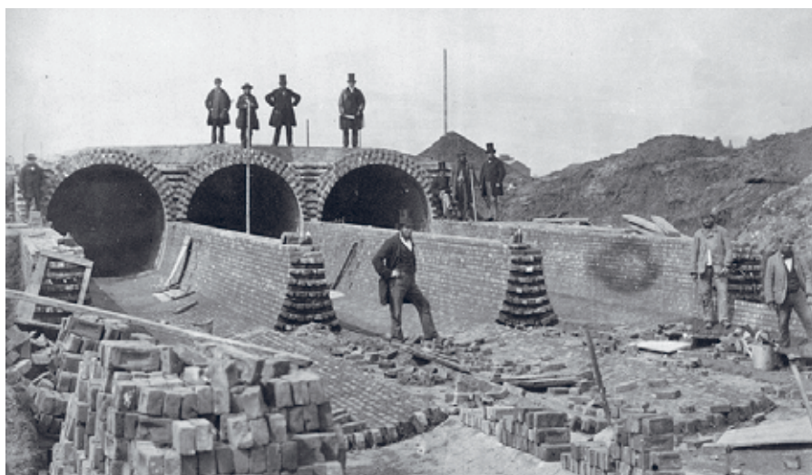
Bazalgette (top right on the bridge) overseeing construction of the sewers
