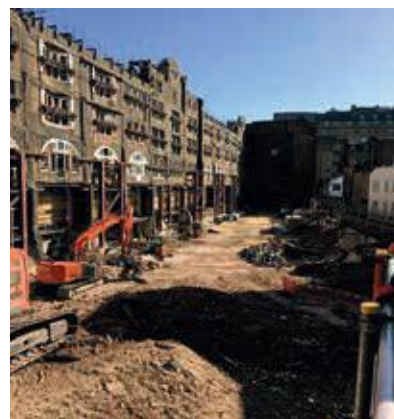
View of the demolition behind the retained façade
