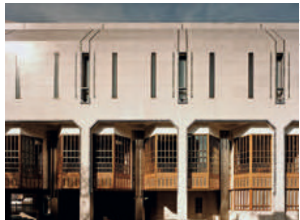
Detail showing windows and panels in stainless steel, teak and bevelled glass, with three different surface finishes to the granite.
