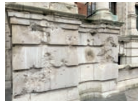
THE DAMAGE TO THESE WALLS IS THE RESULT OF ENEMY BOMBING DURING THE BLITZ OF THE SECOND WORLD WAR 1939-1945 AND IS LEFT AS A MEMORIAL TO THE BRITISH NAVIES OF THIS GREAT NATION AT THE TIME OF COMPLETION
