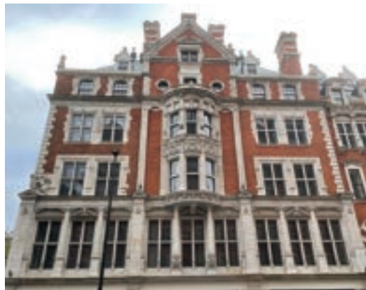
The north east façade.
