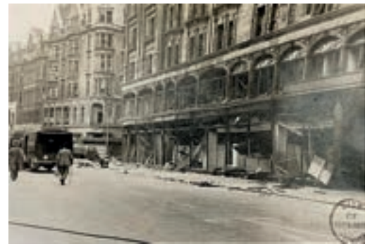
Blast damage at Harrods
