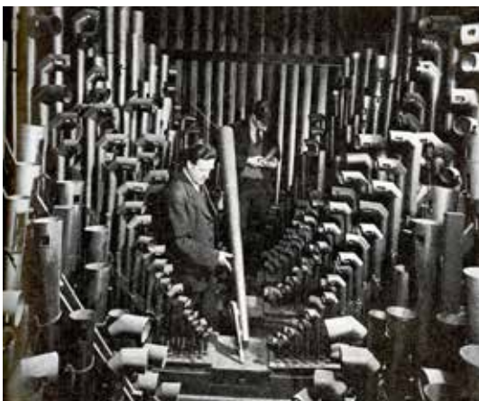
Organ pipes being refurbished, 1974
