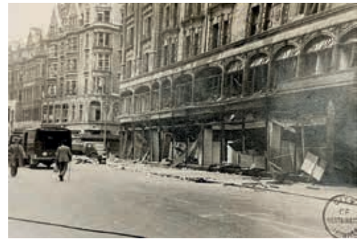
Blast damage at Harrods
