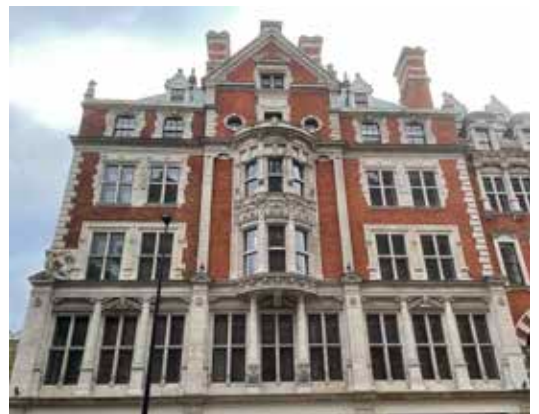
The north east façade.
