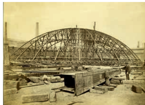
Royal Engineers work on the construction of the dome
