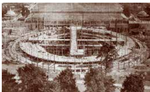
The construction of the Hall
