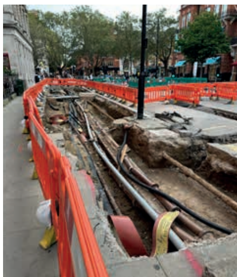
Sloane Street roadworks
