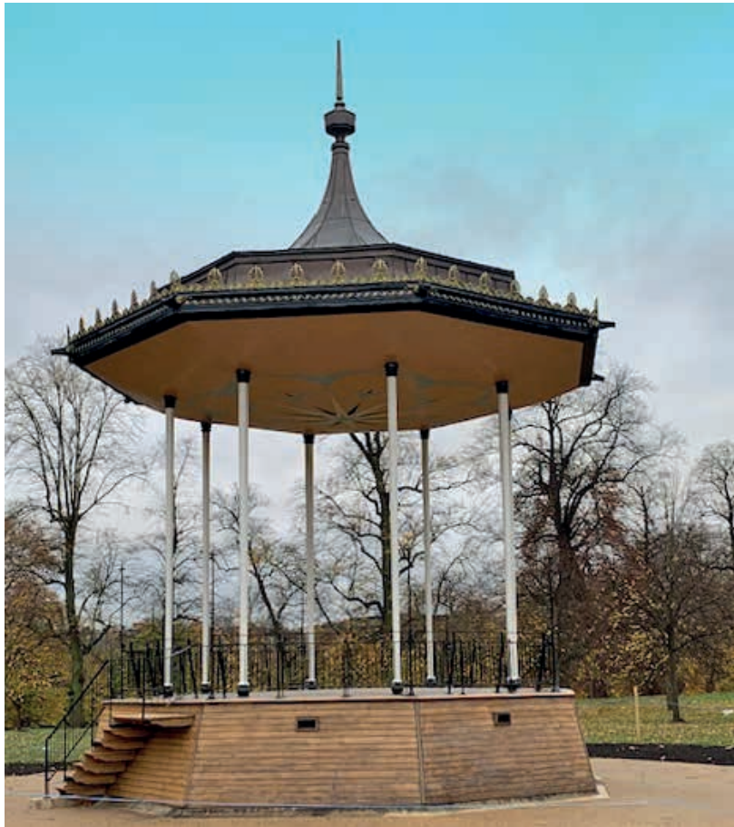
Beautifully refurbished Round Pond bandstand
