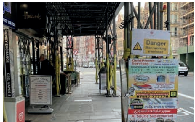
Princes Court scaffolding
