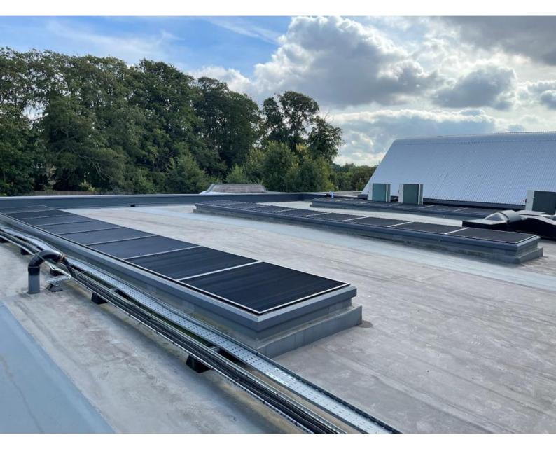
Koolshade<sup>®</sup> provides up to 100% perfect solar shading but with an incredibly 80% open area for near perfect vision, daylighting and natural ventilation.
